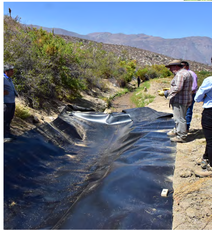
Aguas Claras, Araya, Carachas Canals: Canal liners with geomembrane in various widths and lengths.
